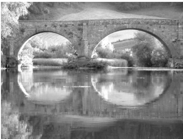
Kerne Bridge – Photo by John Daniels
